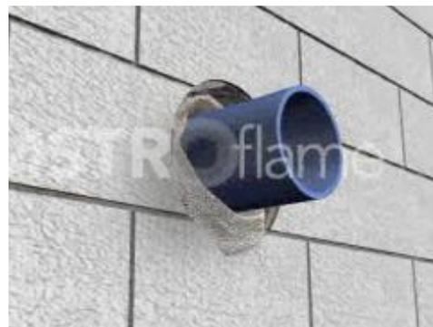
3. Apply HPE to the remaining space around the penetrations. The sealant should be installed at a ratio of 1/8 of the diameter of the penetration, with the maximum diameter being 125mm. (See table below).
