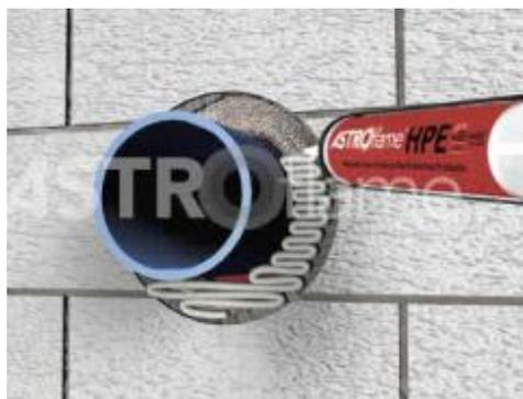
5. Once HPE has been installed to the specified depth smooth over the seal with a spatula dipped in water. Leave the seal for a minimum of 48hrs.
